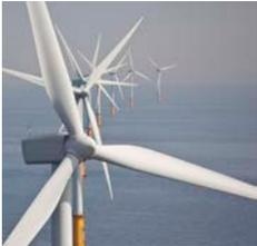
Wind power currently accounts for approximately 24% of the world's global renewable installed capacity. An average wind turbine is comprised of 80% steel, used in the tower, nacelle and rotor.
