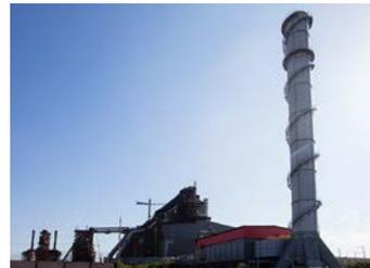
thyssenkrupp has equipped its Duisburg sinter plant with one of the largest fabric filters in the steel industry. The filter reduces dust emissions by 99.99%. It is made up of more than
