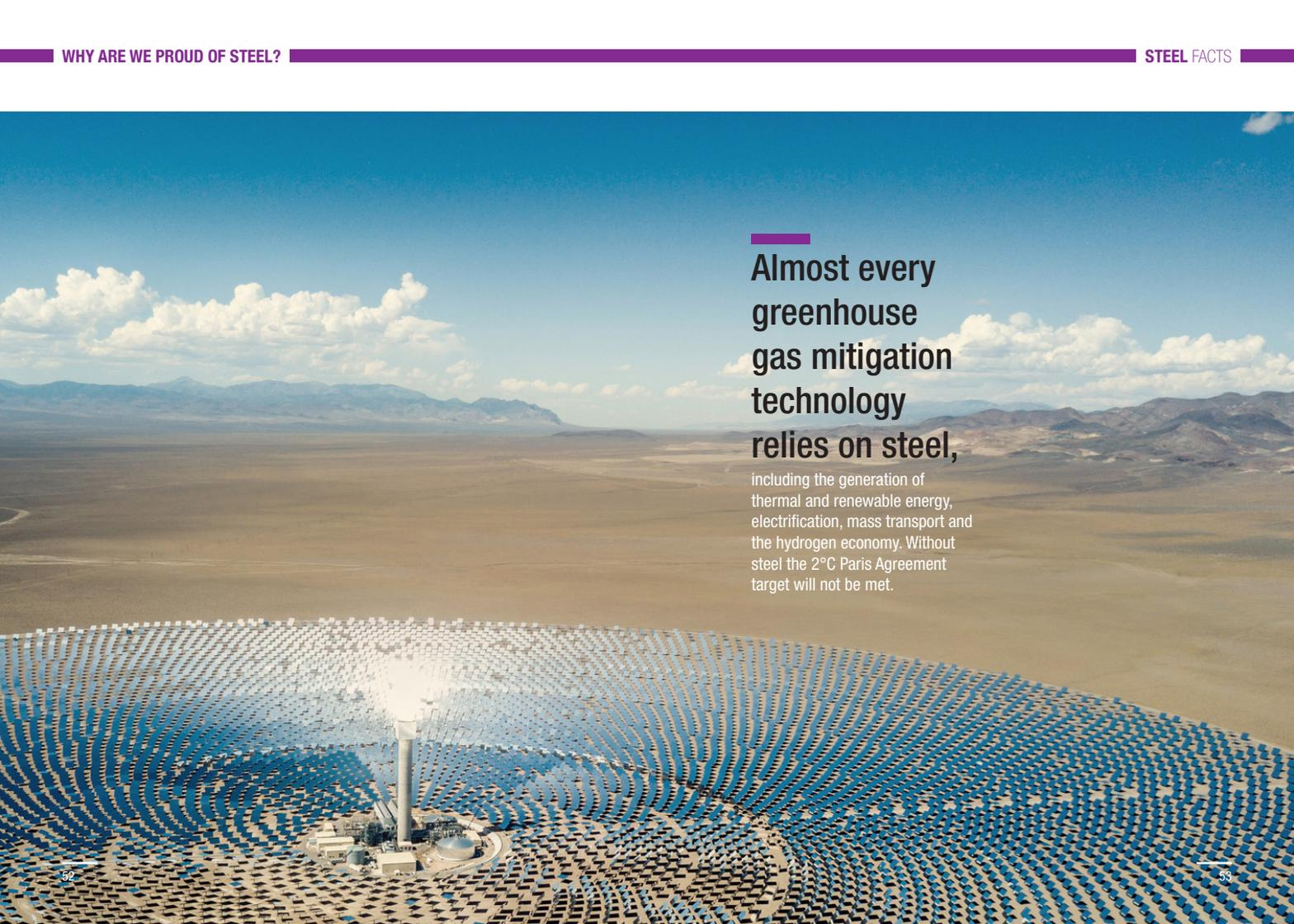
An aerial photograph of a solar tower power plant. The central feature is a tall, white cylindrical receiver tower. Surrounding it are thousands of heliostats (mirrors) arranged in concentric, curved rows, all reflecting sunlight onto the tower. The landscape is a vast, flat desert under a clear blue sky with scattered white clouds. In the distance, a range of low mountains is visible.
